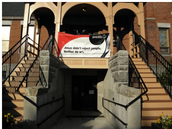
New accessible entrance from the outside. The banner reads, Jesus didn't reject people. Neither do we.
